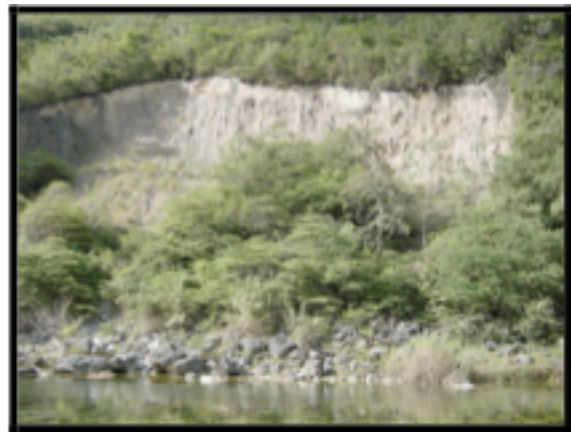
This place is called Chupadero. This whole was made by water leaks from the tunnel from the dam. People are afraid to live in Agua Blanca (41)
