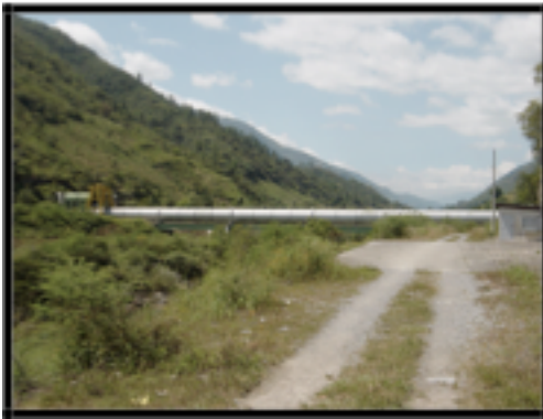
To protect the tunnel of adduction INDE invaded fertile lands and closed access to the communities of the area (11)
