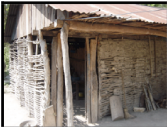
Dña. Nieves de la Cruz house. Most houses are in bad shape due to lack of economic resources and construction materials. (02)
