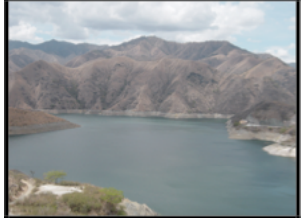
The river's fertile plains were located 100 meters below the reservoir's center.
