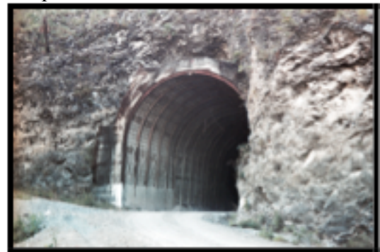
The tunnels built by INDE for vehicles and for water were built on La Campana lands.
