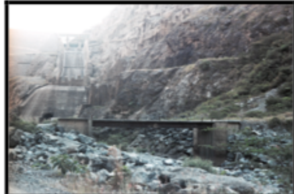
When the plugs are opened, the bridge floods on both sides so it is impossible to cross over to the other side.
