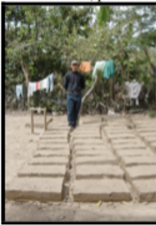
Victoriano Diaz makes adobe for building construction
