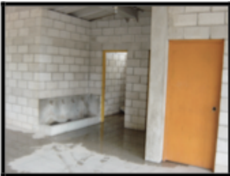
The community hall floods. The pipes are broken. The windows are also broken. It is very small.
