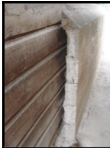
The cement blocks that form the base of Mr. Anastasio Osorio's house have separated.
