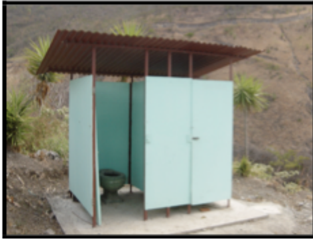
The San Cristobal Parish supported the construction of the school's latrines.
