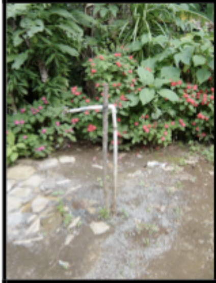
The potable water service needs to be expanded. Water is scarce and does not come in sufficient amounts. Mr. Santo Sucup's water faucet.
