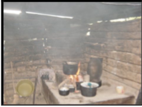
The stoves INDE provided for the houses are not well-built. They are deteriorating. Mr. Alfonso Hernandez's stove.
