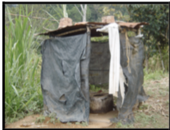
The few latrines built with INDE support are in terrible shape. Mr. Rodrigo Sucup's latrine.
