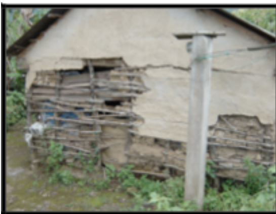
The INDE built houses are deteriorating. Mr. Santos Sucup's house.
