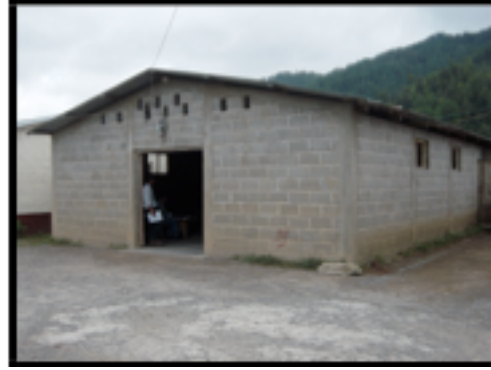
The community hall's roof is deteriorating. INDE did not fulfill its promises.
