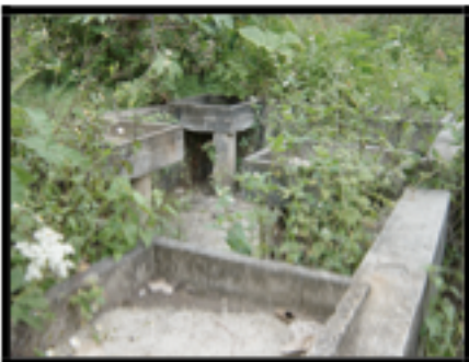
The pila built by INDE was not useful.
